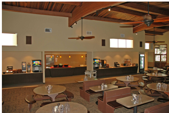
Dining Hall Remodel
